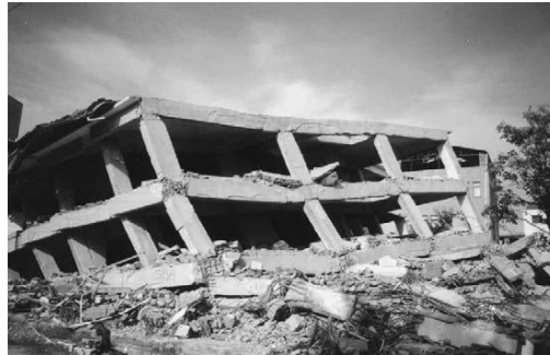
Fig.1 Beam column Joint fails due to shear failure in Kocaeli Earthquake
